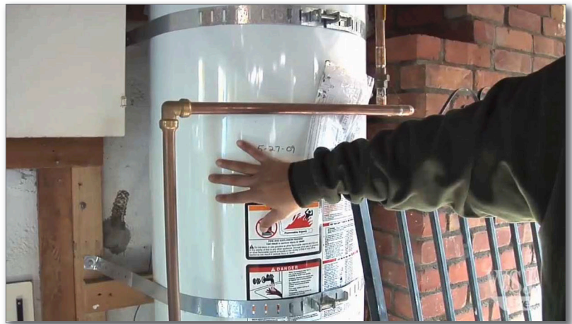
Bricks, wrought iron gate, and a four-year-old water heater are among items to be salvaged during deconstruction. Screen capture from The Wall Street Journal video, "Deconstruction is a growing trend in the West Coast housing market," Dec. 20, 2012. http://on.wsj.com/YrGgX1
