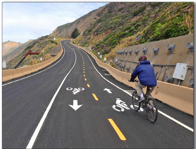
K-rails and bolts. Photo: Andrew Boone, Streetsblog SF.
