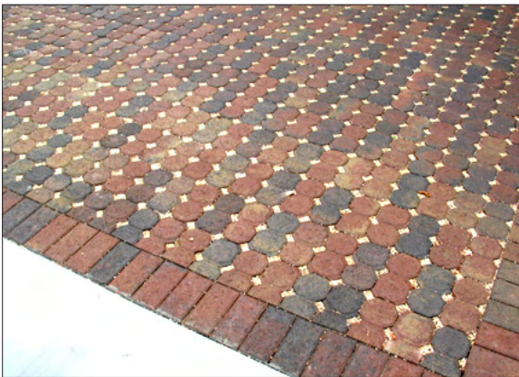
Photo 8: Precast unit pavers capture runoff through openings. Photo: Sarah Sutton
