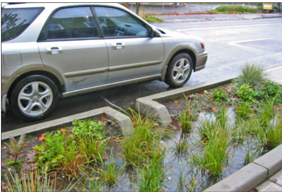
Photos 11 and 12: Portland's "Greenstreets" successfully incorporate rain gardens along roadway parking strips. Breaks in planting allow access to vehicles. Source: Shay Boutillier
