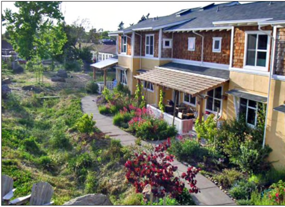
Photo 6: The rainwater leaders from the roof of this multifamily housing unit in Cotati cross under the adjacent pathway and empty into the vegetated swale—a great example of using a physical element, such as a pathway, to separate the neater foundation planting from the more natural (and often weedy) appearance of a drainage swale.
