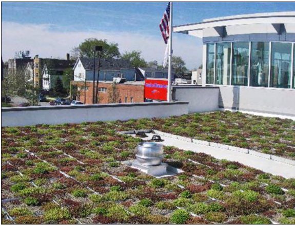
Photo 9: A modular green roof system is a viable alternative to custom installations. Source: www.greenroofblocks.com
