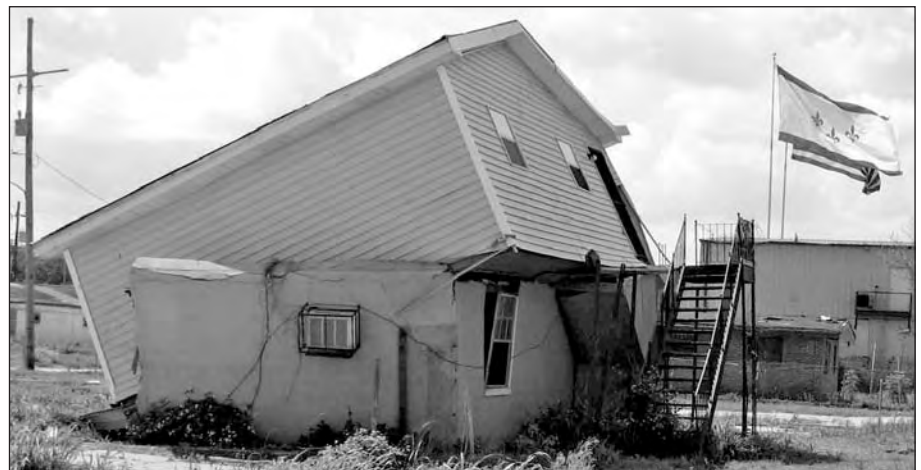
House, Lower Ninth Ward, New Orleans, March 2007
