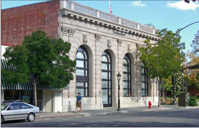
Downtown Livermore mobile workshop—Bank of Italy
