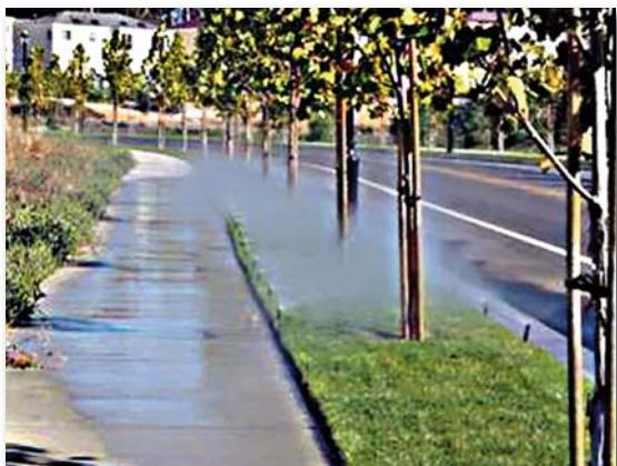
**Figure 3.** Spray irrigation in narrow turf parking strips will always spill over onto adjacent paving, wasting water and reducing life of pavement.
