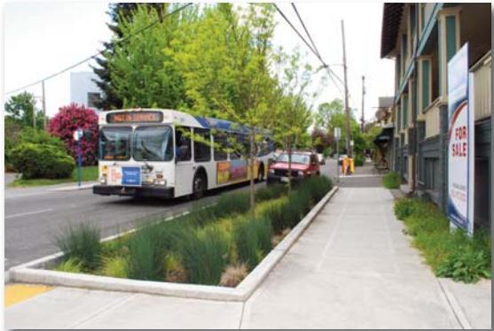
**Figure 2.** Portland Rain Garden. Road runoff flows through curb cuts into curbside planters. Raised curbs and linear planting of sedges, rushes, and trees offer a formal, urban appearance. Photo: Sarah Sutton
