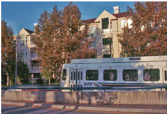
San Jose light rail train passes in front of Ryland Mews. Because it is located close to a transit stop, the developer was able to reduce the number of parking spaces and increase the number of apartments. The higher density created moderately priced apartments in the middle of high-cost Silicon Valley. Photo courtesy of the Local Government Commission.
