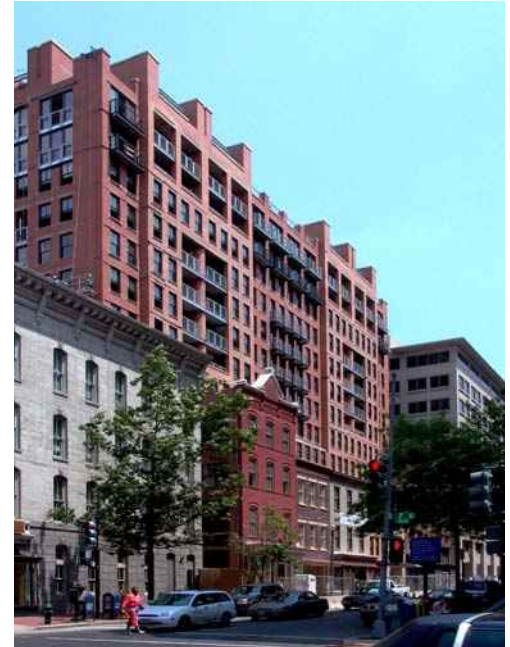
New condominiums rise in the historic Penn Quarter, bringing Washington, DC closer to its goal of adding 120,000 new residents by 2025.
