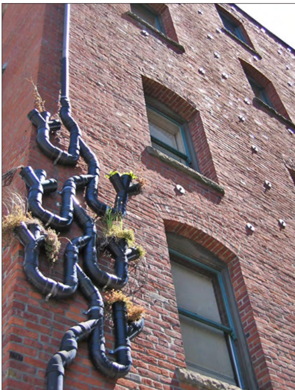
Photos 18: Creative modification to a standard downspout slows roof runoff
