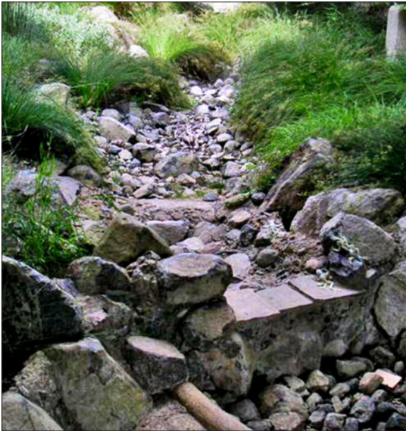
Photo 15: This infiltration trench with a cobble bed, lined along the perimeter with fine textured grasses to filter sediment and pollutants, remains an attractive arroyo-like landscape feature during the dry season. Source: Marc Richmond, Practica Consulting
