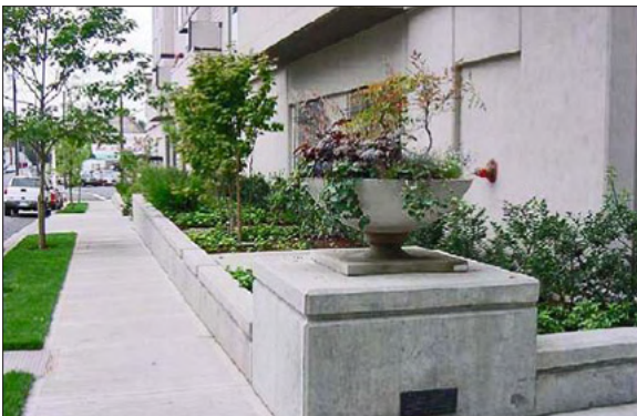
Photo 10: Flow-through planter. Source: City of Portland 2004 Stormwater Manual
