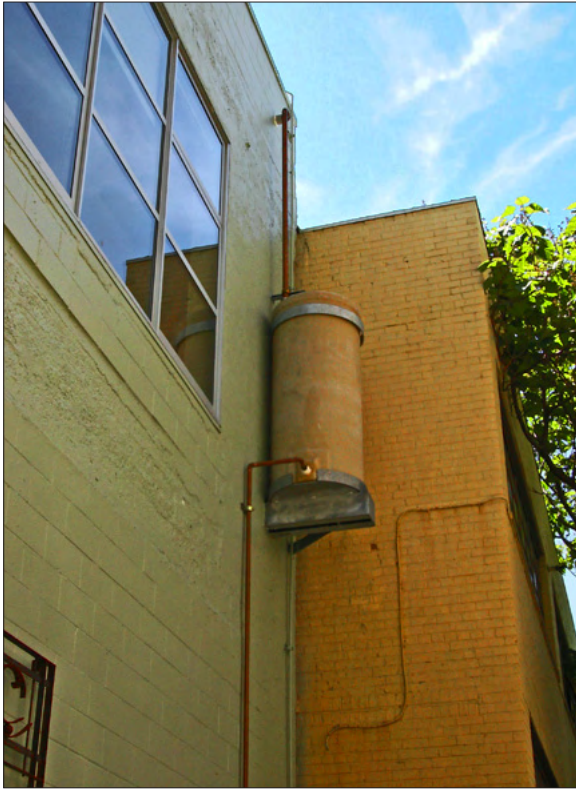
Photo 17: Cistern attached to the outside wall of StopWaste.Org headquarters in Oakland
