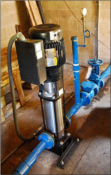
Newly installed electric water pump
