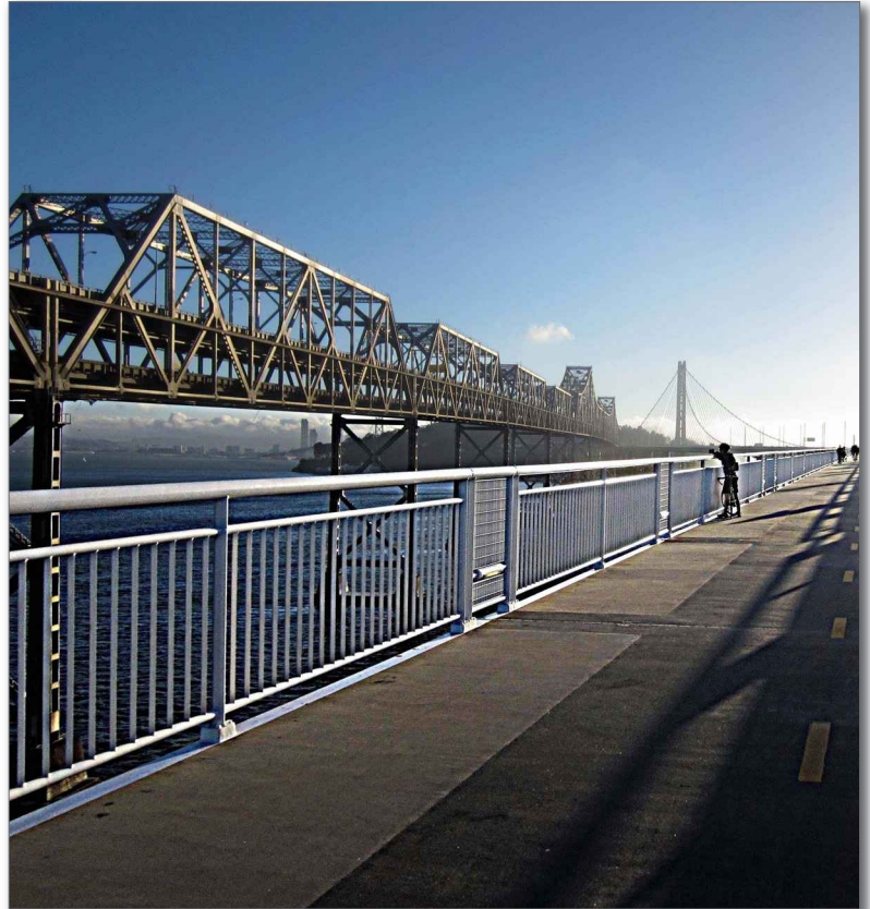
Looking southwest at the abandoned cantilever span.
