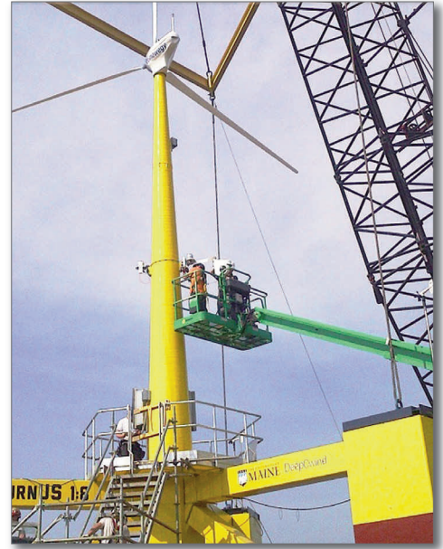
Workers prepare to launch VoltturnUS 1:8. Source: U.S. Department of Energy
