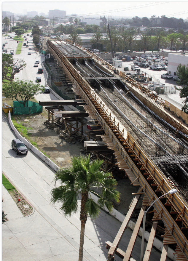
Expo Light Rail Phase 2 construction. Looking east toward Bergamot Station, May 2013. Olympic Blvd. at upper left. Image courtesy of Expo.
