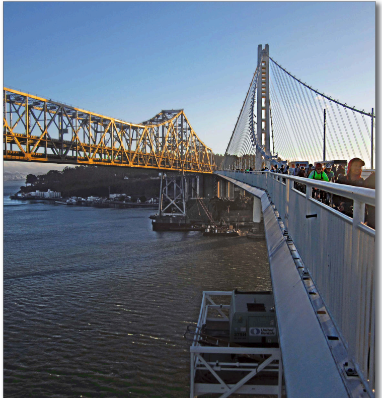
Looking southwest at the old and new eastern spans. Photo © Jonah Chiarenza, AICP
