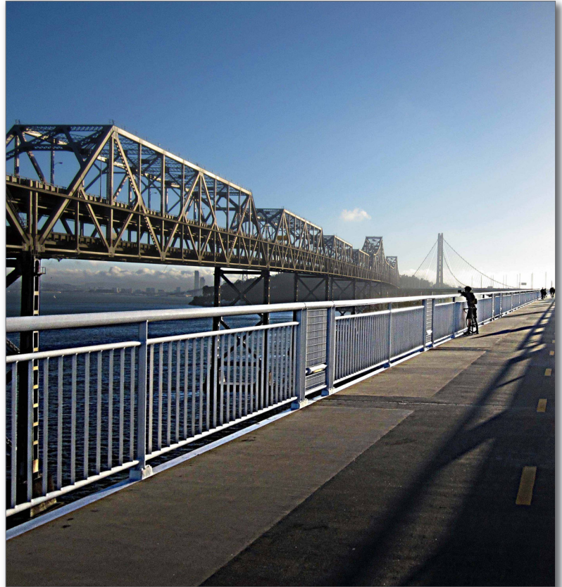
Looking southwest at the abandoned cantilever span.
