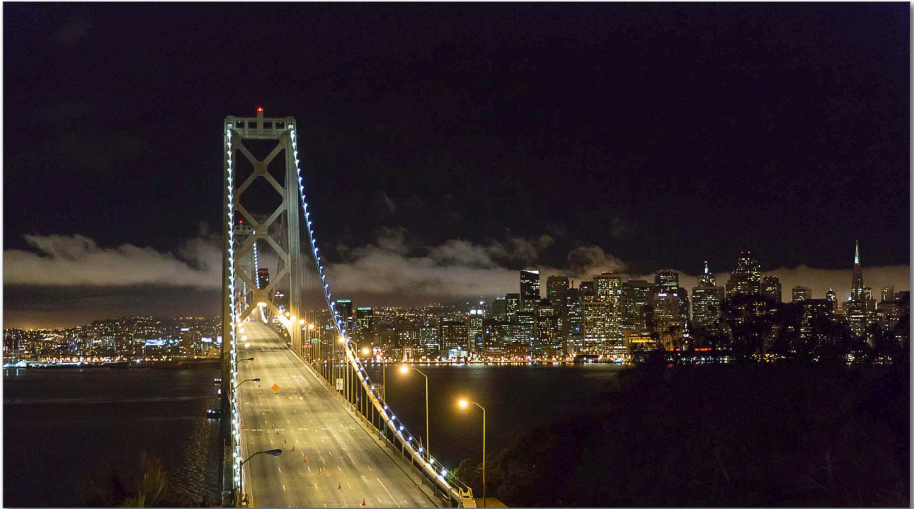
Above the existing western (suspension) span at night, looking southwest to San Francisco. Photo © James Pan ■
