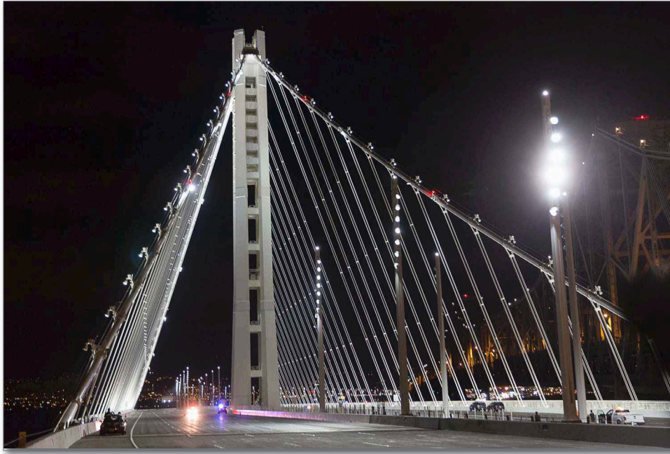
New tower and cables, seen from the roadway. Photo © James Pan
