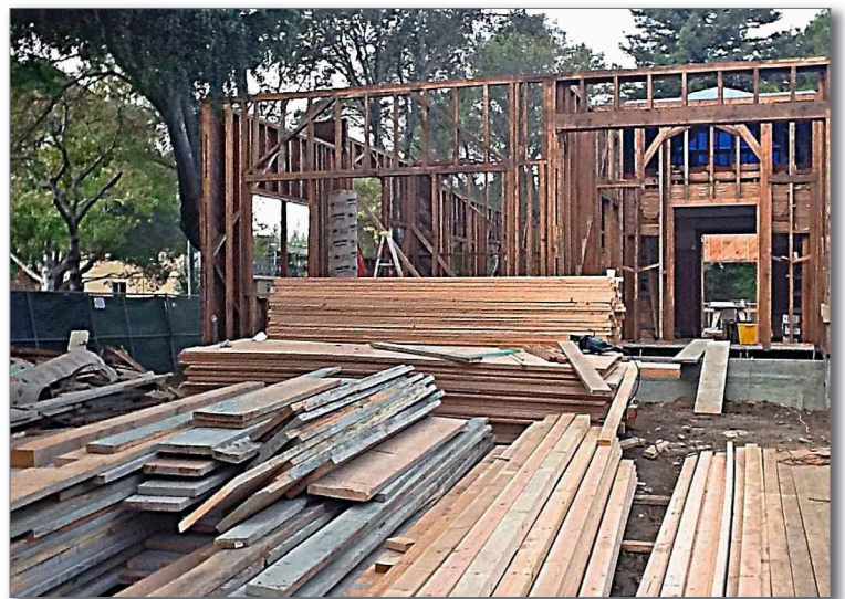
The original first floor framing of this deconstructed house remains in place on a new foundation, January 2014. Recycled lumber on the left is from a different house. Photo: Naphtali H. Knox, FAICP.
