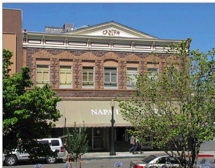
The Center Building (1904), 816 Brown St. Constructed of rough-cut native stone and brick, this is one of only a few stone buildings remaining in the city of Napa. "The decorative stone trim of the windows is a major feature with quoins and radiating stones at the window heads in a contrasting color accenting the windows."
