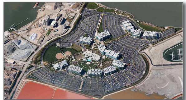
Pacific Shores Center, Redwood City. Credit Google Maps
