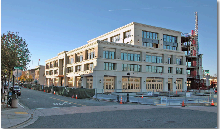
The new Taylor Farms neoclassical building in downtown Salinas — almost completed, and just beautiful. Photo courtesy Belli Architectural Group, Salinas.
