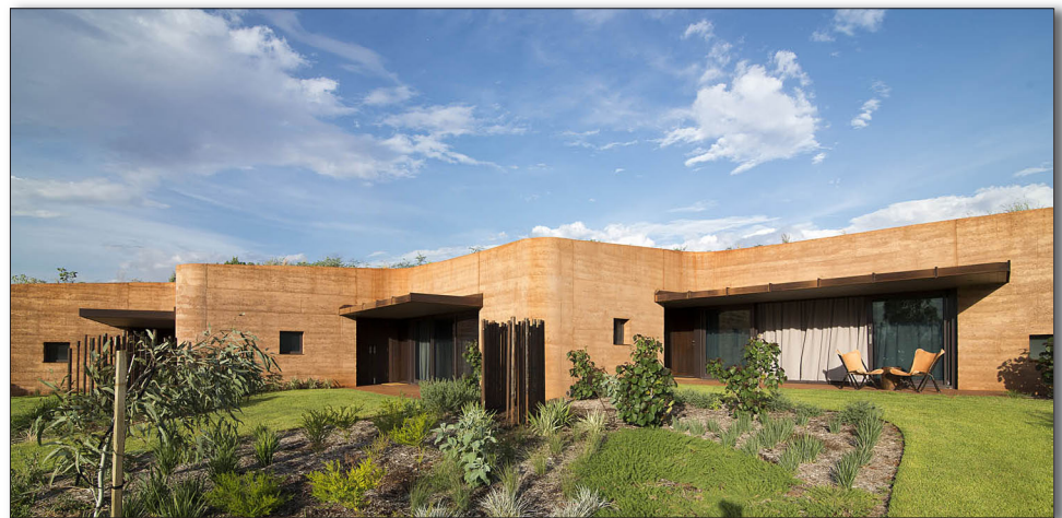
The residences — contiguous but not internally linked — are stepped to maintain privacy on each covered veranda. The rear walls are buried under the sand dune. Courtesy Luigi Rosselli Architects © Edward Birch
