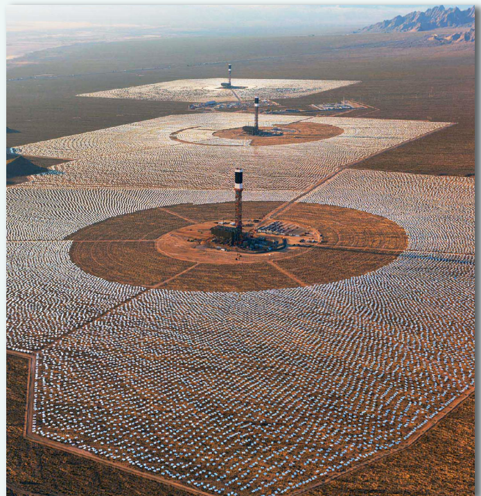
Utility-scale solar. The Ivanpah Solar Electricity Generating Station in the Mojave Desert. Photo courtesy of Brightsource Energy.
