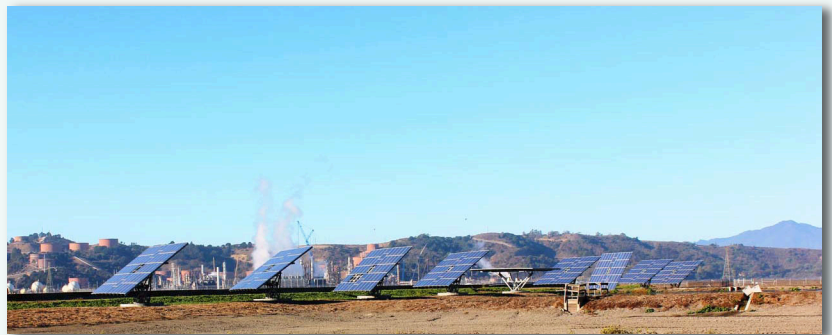
Distributed generation. Solar panels at the West County Wastewater District collection and treatment facility, Richmond. Photo: Josh Hohn.
