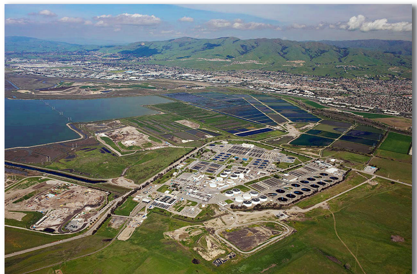
Aerial view, San Jose-Santa Clara Regional Wastewater Facility. Photo: City of San Jose.
