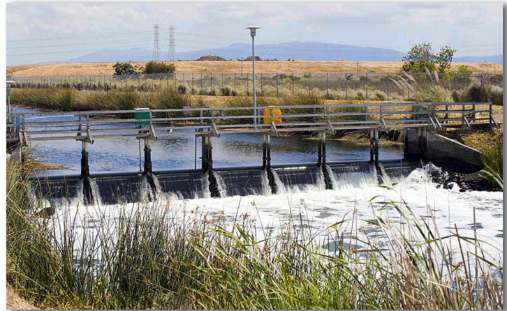
Treated effluent from the San Jose-Santa Clara Regional Wastewater Facility entering the Artesian Slough, which eventually flows to the South Bay. Photo: City of San Jose.
