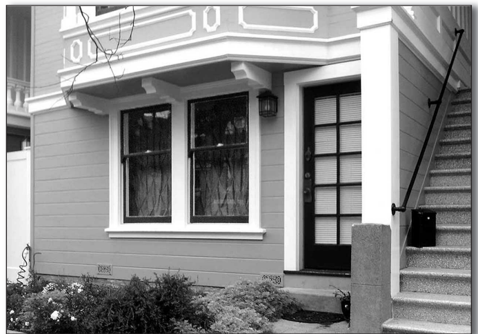
A completed dwelling unit replaces the ground floor basement and garage. Credit: APA
