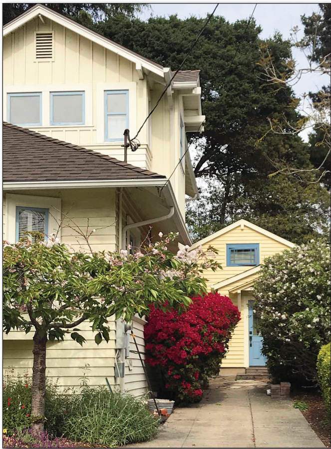
A garage converted to an ADU southwest of the Claremont Hotel. Photo: Denise Pinkston
